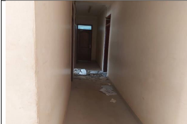
Corridor at Level 2 before works
