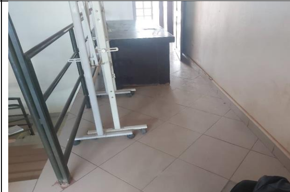
Foyer at level 2 before works
