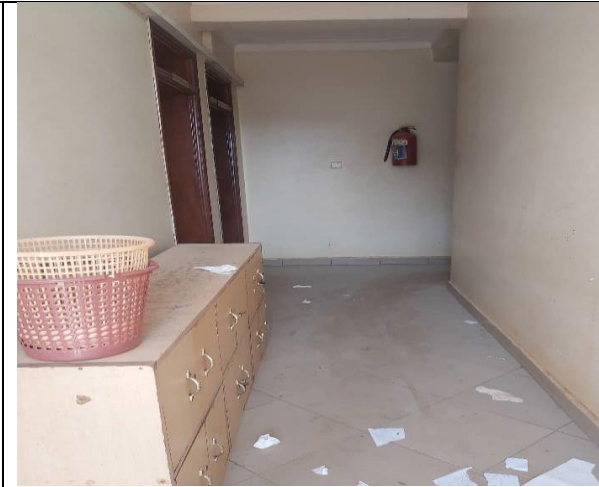
Corridor at Ground floor before
